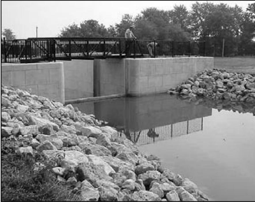
Lock 14 North, located 5 miles North of St. Marys West of St. Rt. 66 on Lock 14 Rd, now boasts a pedestrian bridge on the upstream end of the lock, stone parking lots on the towpath and sidespillway sides, landscaping, seeding and bank protection.
