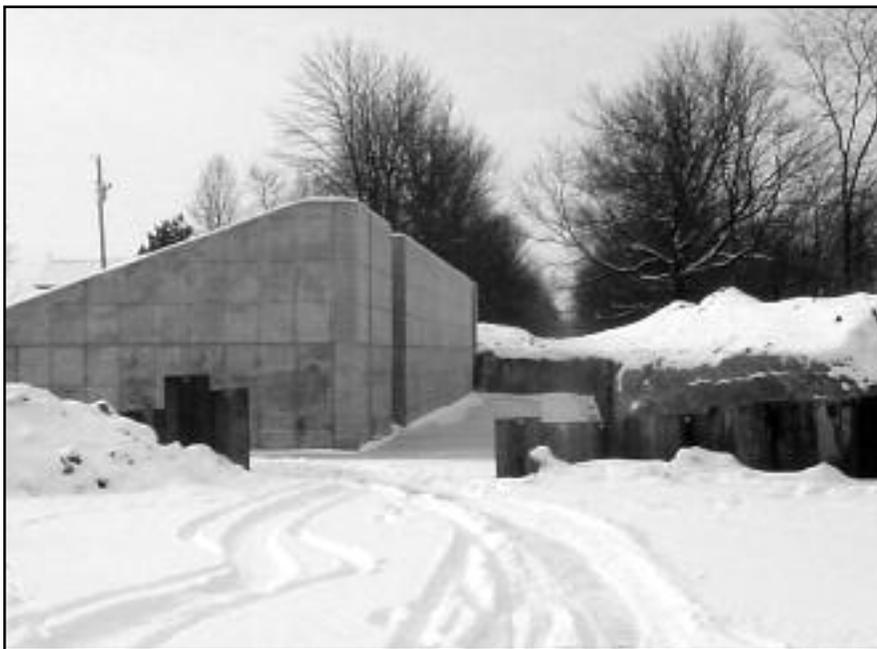
**THE NEW LOCK 14** -- Lock 14 is being refurbished with new concrete walls. The project was halfway done before cold weather postponed completion until spring. The project is part of Phase II Canal Improvements by the ODNR Division of Water.
