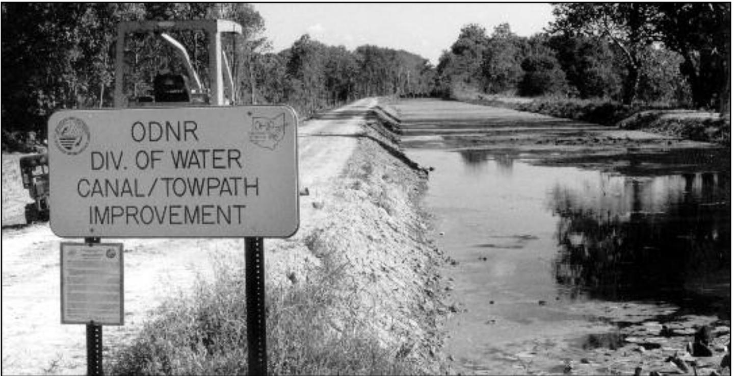
***Funded partially by a federal grant, ODNR is making major improvements to the canal bank near Kossuth. The project objective is to reinforce the towpath where the canal is “above ground.”***
