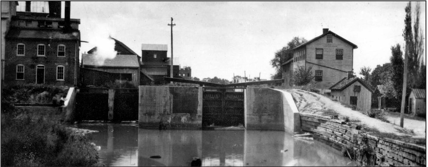
*Photo of Lock One in New Bremen shortly after it was converted from a wooden lock to a concrete lock. This is one of many photos being gathered to include in a book MECCA hopes to publish about the Miami-Erie Canal.*
